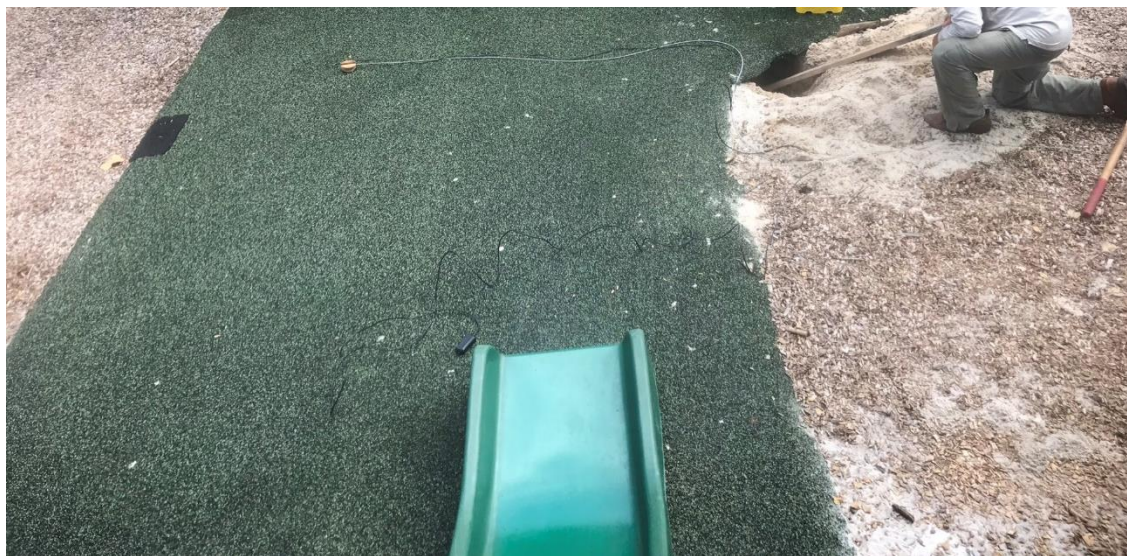
Figure (10)- Scope and excavation at location ID-3
