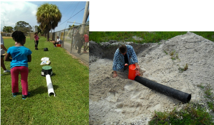
Artificial Burrow with Industrial Control Valve and Ernest's Perforated Pipe and Bucket Burrow
